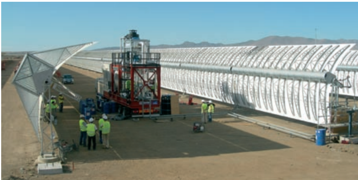
Installation of SENERtrough collector system at Andasol 1 solar plant.
